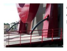
Close up of curved gear rack for the Red Bridge draw bridge manufactured by SANDERS, the Netherlands.
